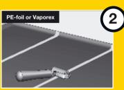
If the moisture content of the sub-floor is higher than 1,8CM% but less than 5CM%, always use Grabo Vaporex damp-proof underlay floor. If the moisture content is less
